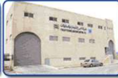
Warehouse and CAC in Amman (Sahab) - 1999
